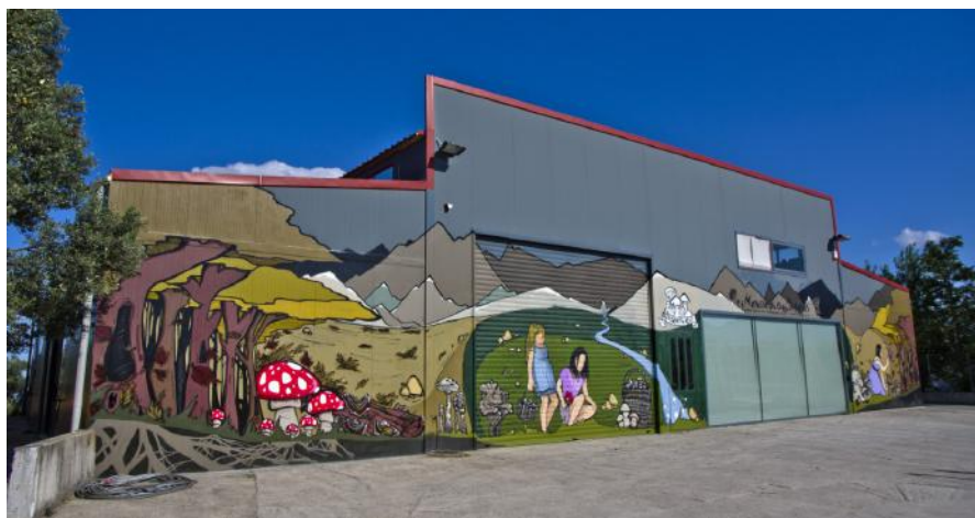
Dirfis Mushrooms - exterior view of the packaging plant, photo : Dimitrios Malliaris
